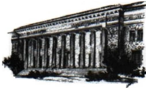
Tehama County Courthouse
