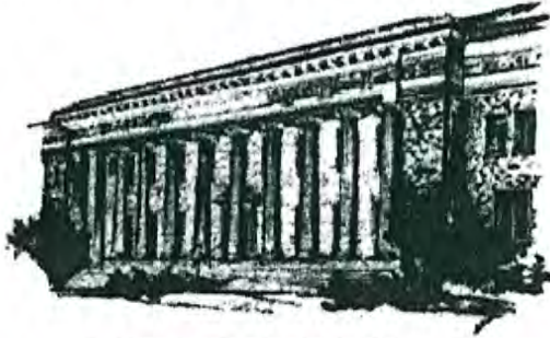
Tehama County Courthouse
