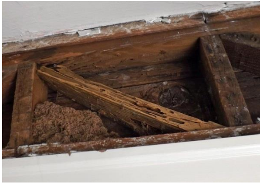
Carpenter ant damage on a structure
